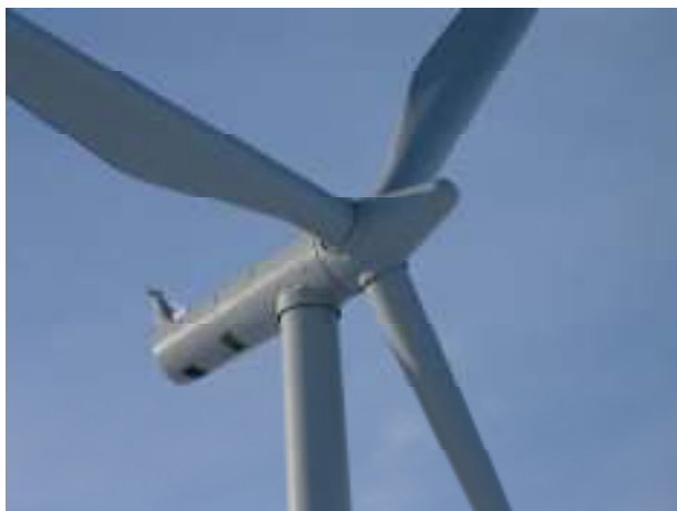
2.0MW Siemens Wind Turbine (above) at Whitelee Wind Farm Scotland
